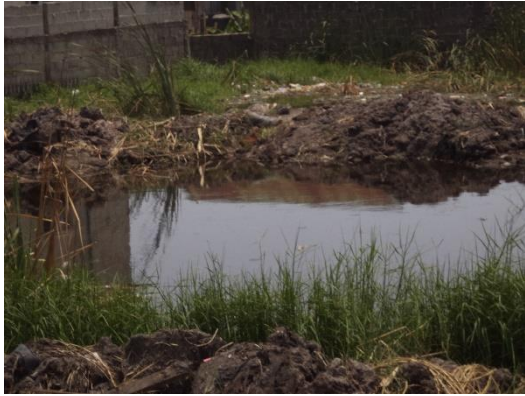
Pic 1: location of repaired Pipeline
